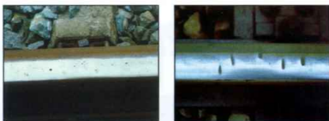
Fig. 5: Ballast stone imprints, small (left) and medium (right)
