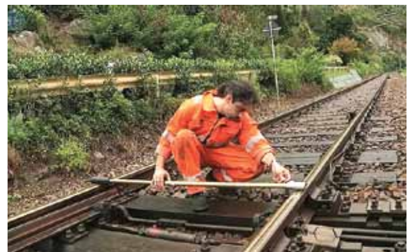
Below: Fig 9. Checking the wear situation at the switch blade.
