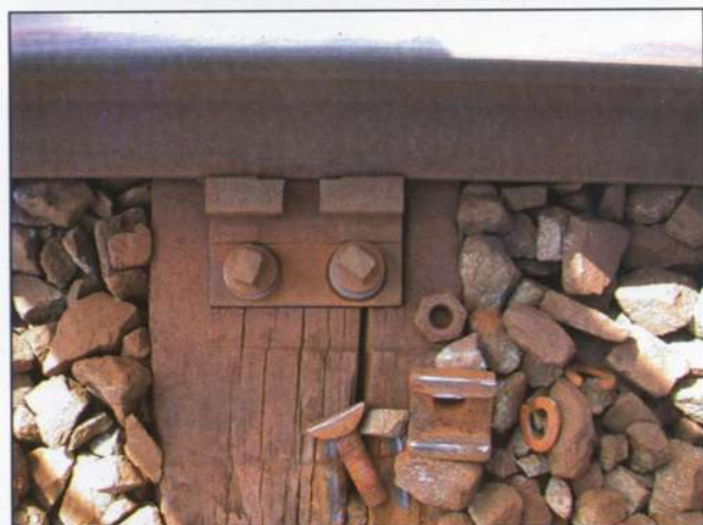
Fig. 3: K-fastenings that have become loose due to rail corrugation
