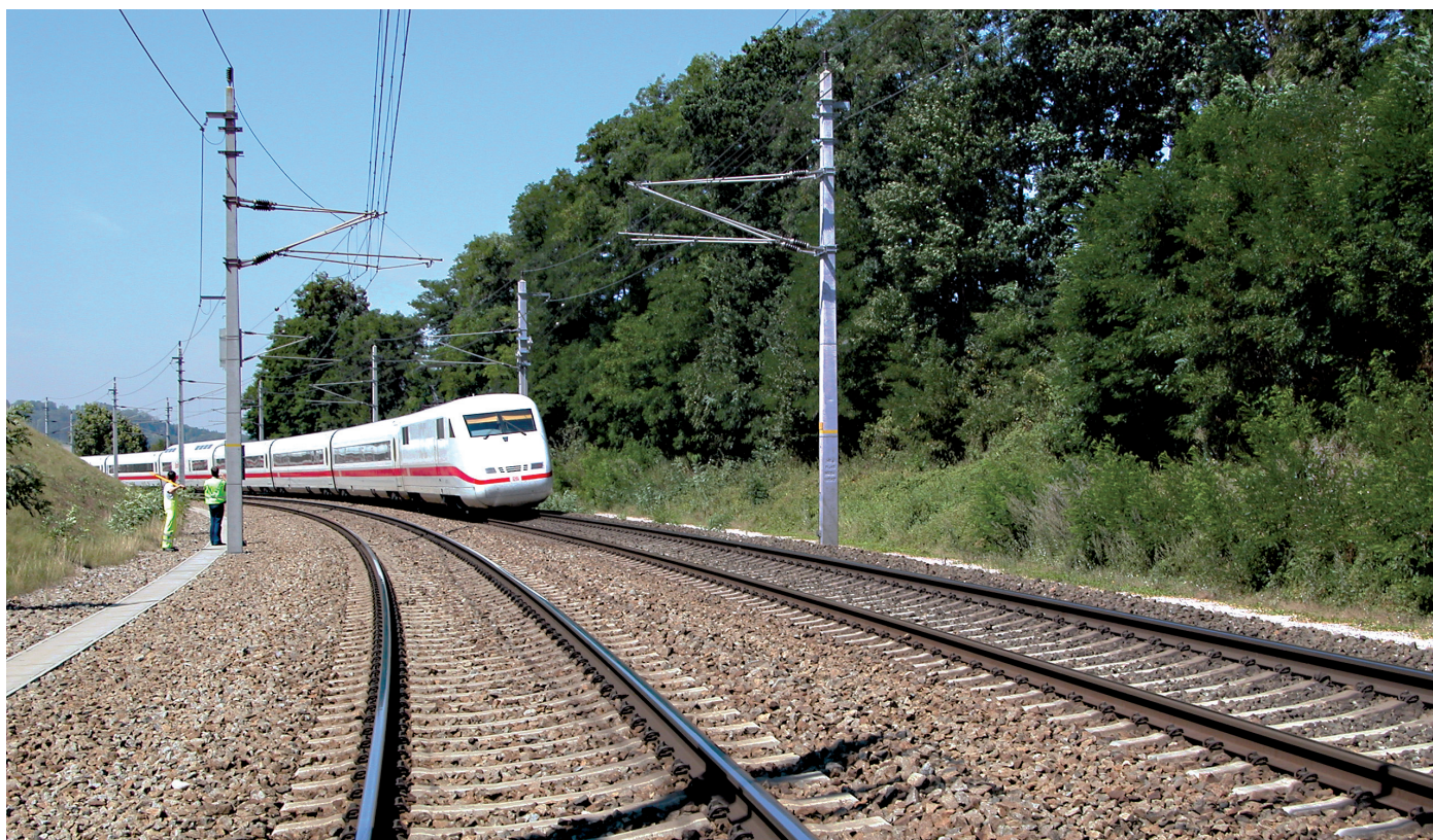
DB Netz has extended the application range for R350HT rail in curves from a maximum radius of 700 m to 1 500 m for intensively-used track.
