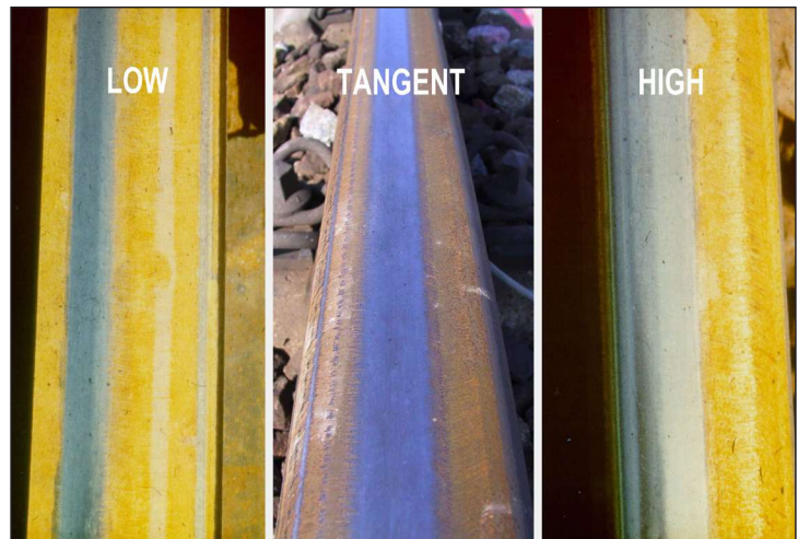
Figure 3. Rail profiles are designed to provide the desired contact geometry on the high or low rails in curves, or both rails in tangent track.
