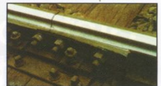
Fig. 5: Lateral wear
