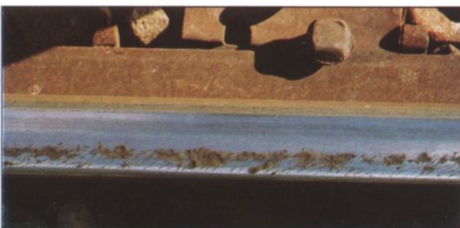
Fig. 5: Rails before (top) and after (bottom) preventative/cyclic grinding
