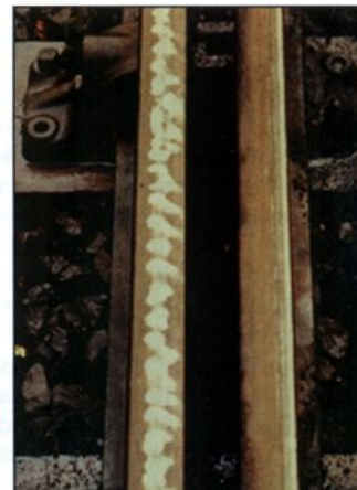
Fig. 11: Short-pitch corrugation
