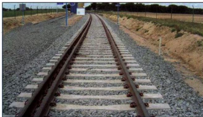
Fig. 16: Spanish double-gauge trial track
