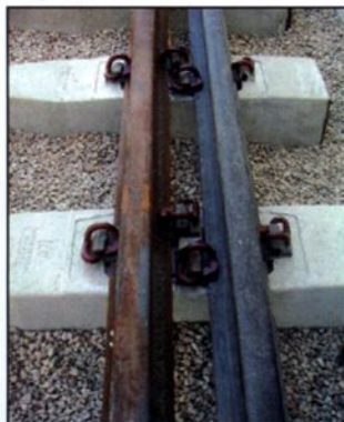
Fig. 17: Example of a fastening system taking up little space (DSA fastening system of Railtech)
