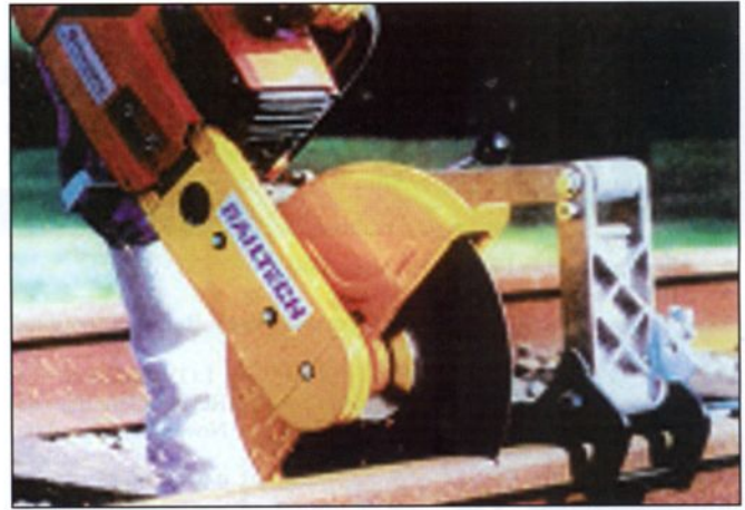
Fig. 26: Rail sawing
