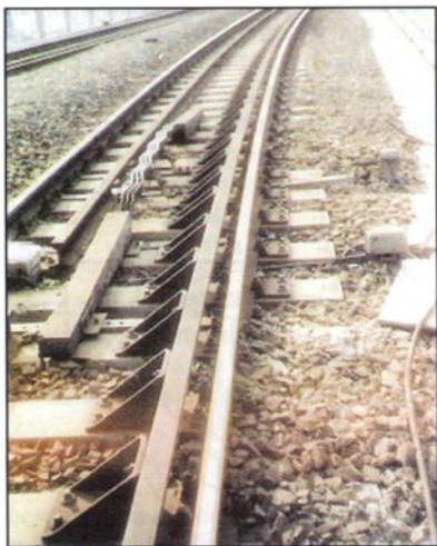
Fig. 19: SNCF RER line C - active guard rail and safety rail
