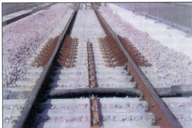
Fig. 21: Expansion joint, SNCF design from 1993/1994
