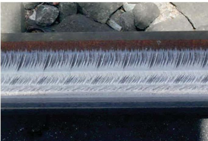
Abb. 7: Geschliffene Schiene – raues (aggressives) Finish
